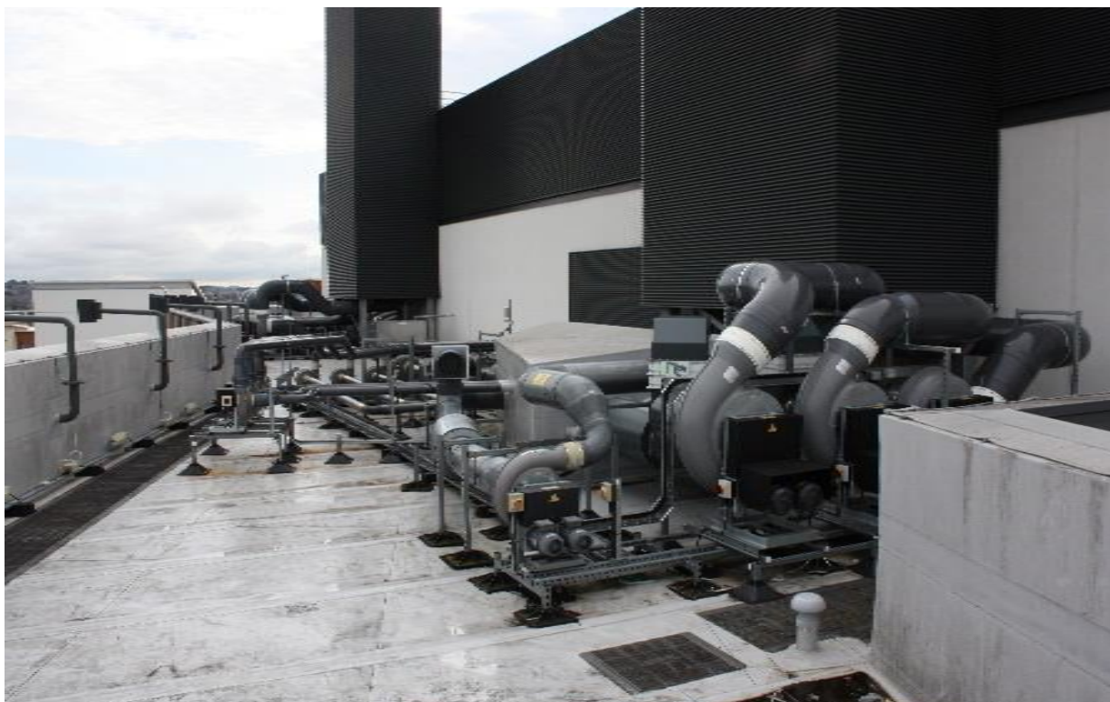
PVC Fume extraction systems to serve fume cupboards
