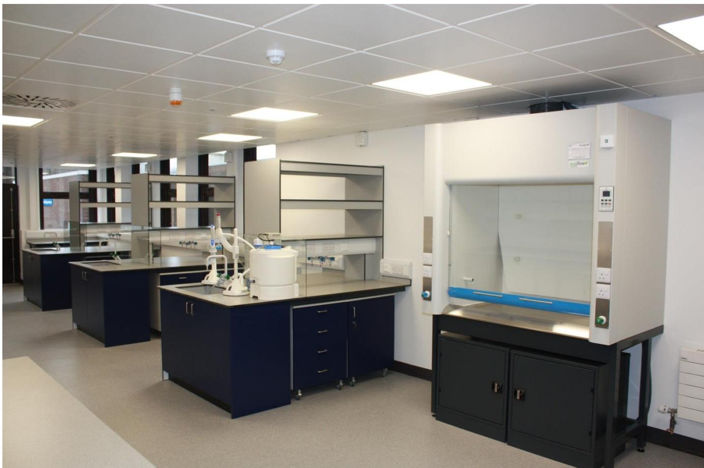
Project Scope – Design, manufacture and install Fume Cupboard, Extract Systems, Supply Air Systems, Laboratory Benches, Service Outlets and Bespoke Sinks.
