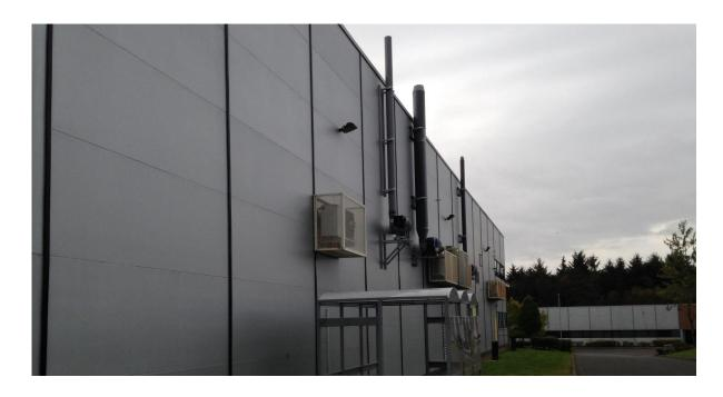
Project Scope – Design, manufacture and install polypropylene extract system, controls and extract fan for specialist lab local extract ventilation header.
